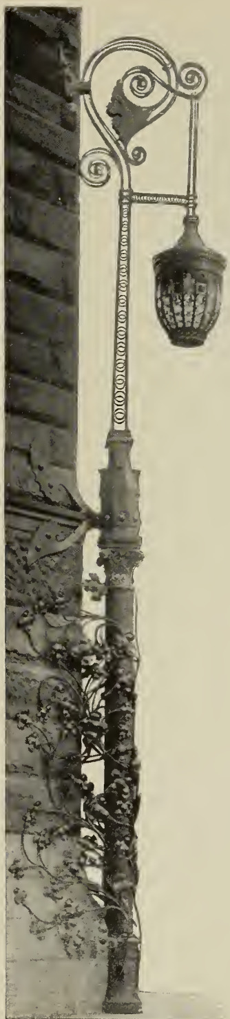
A.—ELECTROLIER, SOCIETY FOR SAVINGS BUILDING, CLEVELAND, O. Wrought Iron, Hammered Leaf Work, Bower-Barffed.
